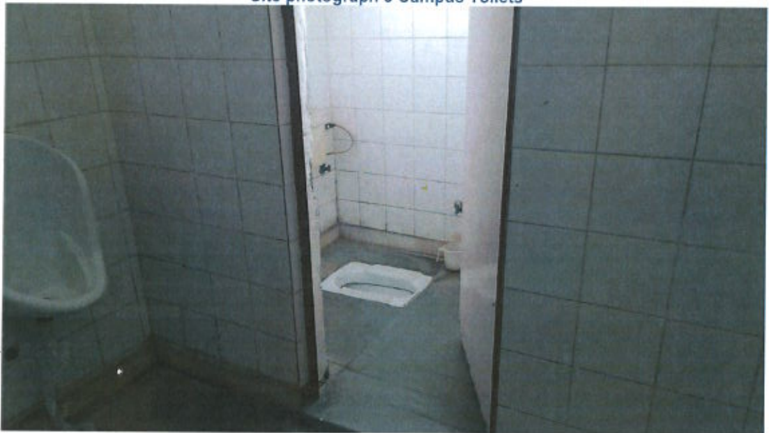
Site photograph 3 Campus Toilets
